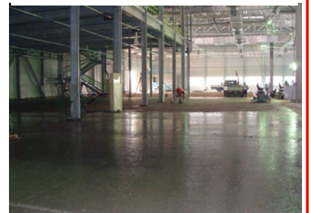
Floor Finishing in progress
