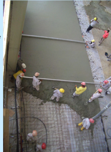
FACE M.E. supervising the construction of DM2 slab
