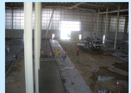
Casting in progress. Most slabs achieved DM1
