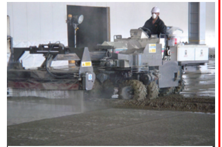
Topping Spreader in action
