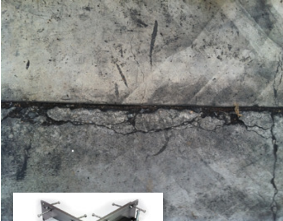
ABOVE: Poor floor joints. LEFT: Armour joint. BELOW: Finished joint repair.
