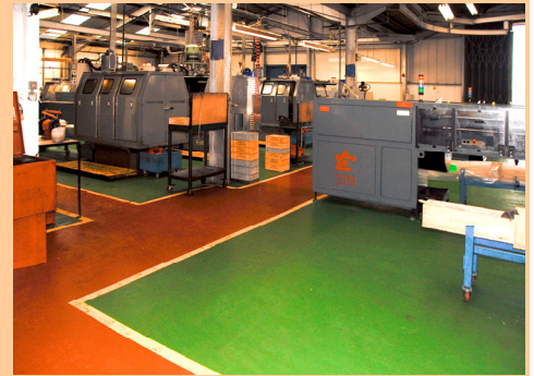
Newly refurbished floor at Tappex site
