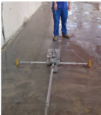
FACE Middle East surveying the proposed aisle ways the day after floor construction, using the FACE Digital Appendix C Profileograph.
