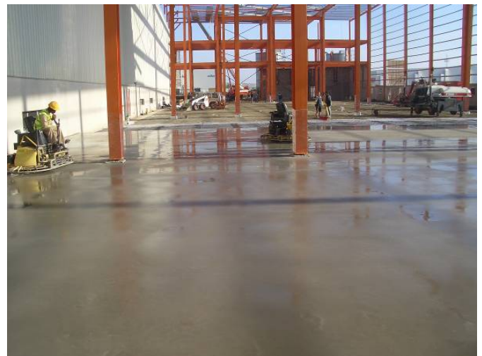
Finishing and preparation for the next floor slab
