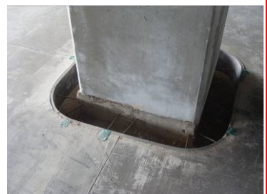
Columns are fully isolated from the slab and backfilled later
