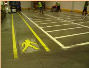
Pedestrian walkway and boxed storage area line marking applications
