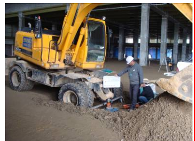
A Plate Bearing Test was done to confirm the Sub-Grade K-Value
