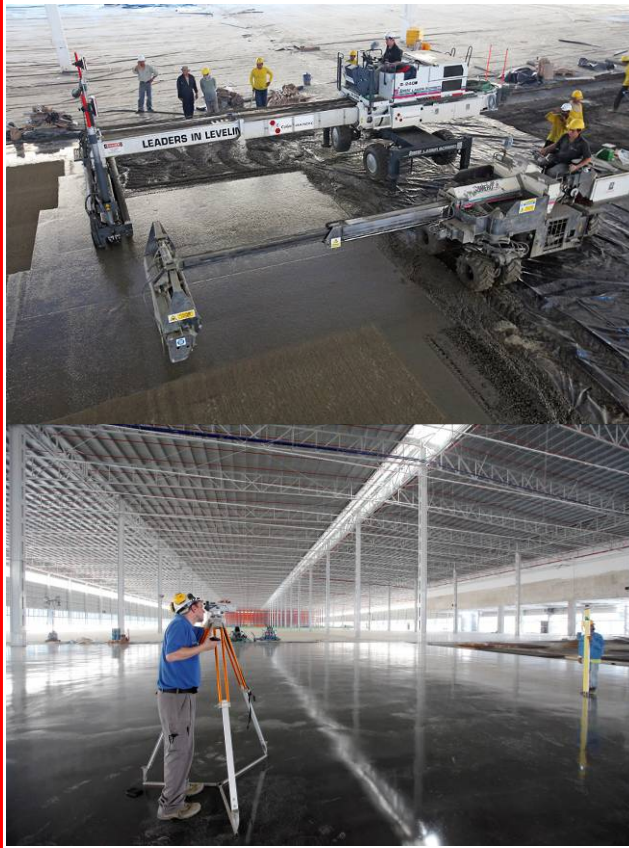
Pictures from top: Construction of a Steel Fibre only SOP. Face Consultants surveying floor.
