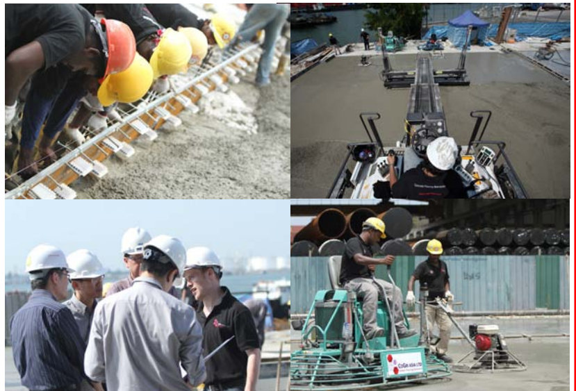
Images from top left: Armoured joints; Laser Screed; Rob Walker talking to visitors; finishing.
