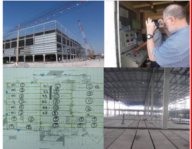
Images from top left: Site in Thailand; checking the concrete mix; pour sequence; precast concrete slabs.
