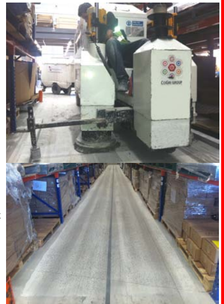
From top: The Laser Grinder® on-site in Australia; Ground aisle.
