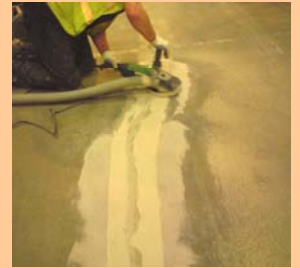
Joint repair in progress
