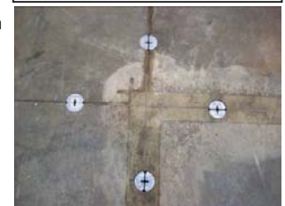
CoGri Joint Stabiliser installed
