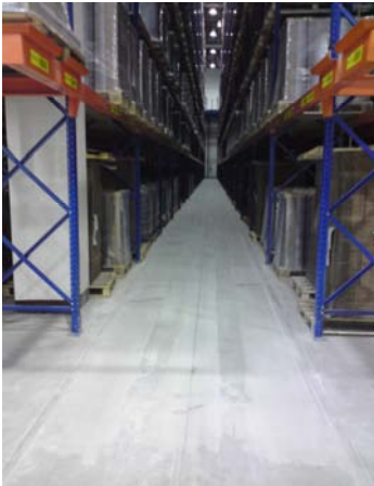
ITTM: 3-Wheel Truck Grinding
